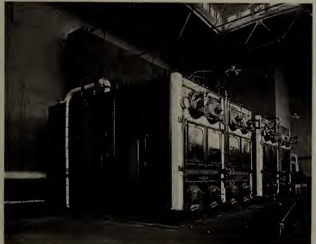
BOILER-ROOM POWER PLANT PORTLAND RAILROAD COMPANY, Portland, Me. Sheaff & Jaastad, Engineers, 85 Water Street, Boston.
